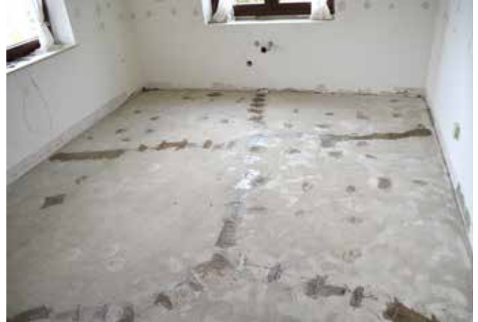
Provision of a flat, clean and dry surface.
