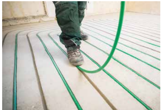
Laying of KLIMAPEX ® heating pipes in the cut grooves.
