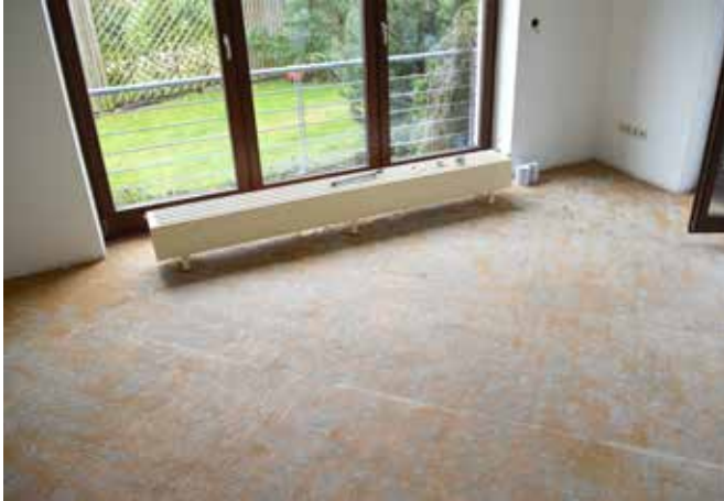
Removal of the existing top layers and radiators.
